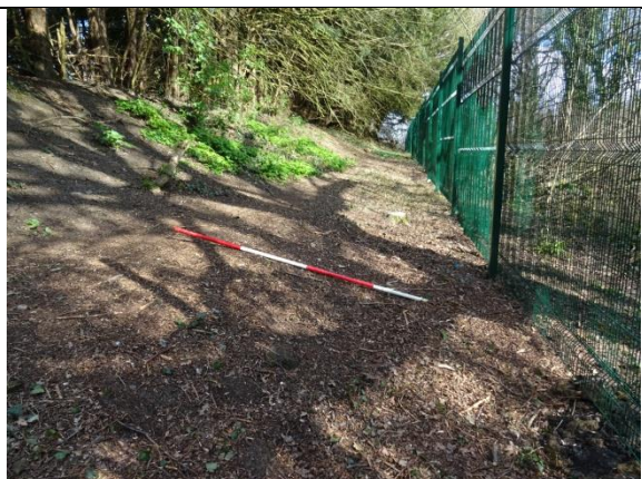
East Side by Post 63 after fencing installed
