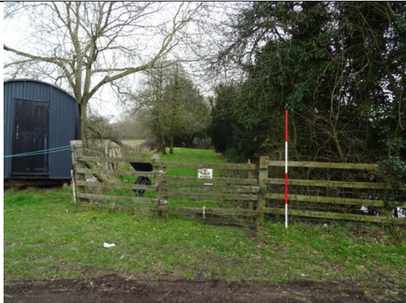
North Side by Post 126 before work
