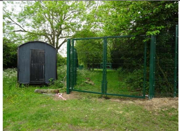
North Side by Post 126 after fencing installed
