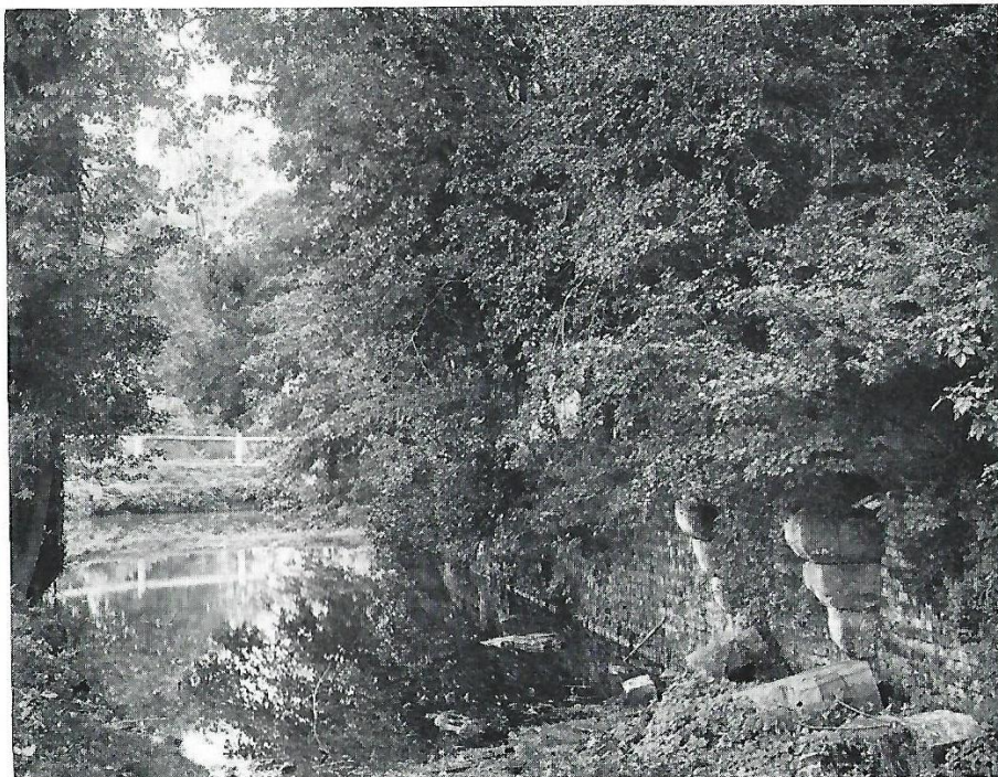
THE MOAT AND RUINS OF DRAWBRIDGE, SCADBURY
