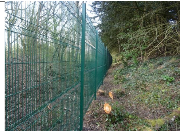
East Side by Post 36 after fencing installed
