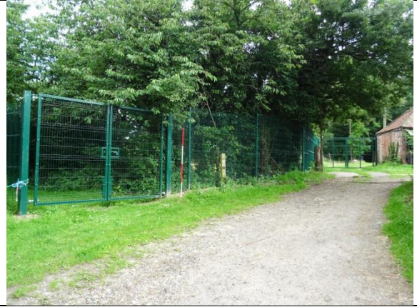
North Side by Post 125 after fencing installed
