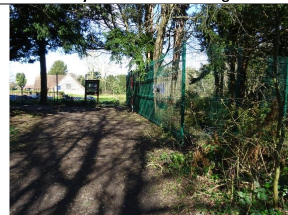
South Side by Post 80 after fencing installed
