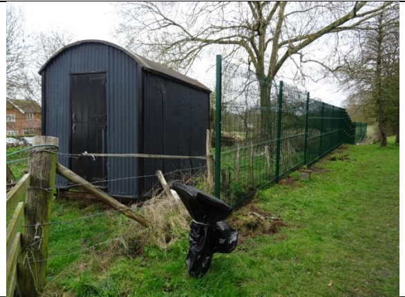
North Side by Post 1 after fencing installed
