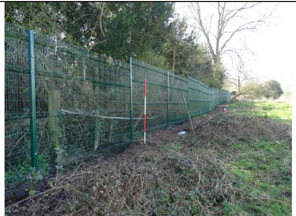
North Side by Post 29 after fencing installed
