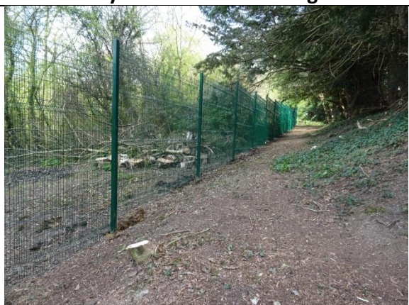
South Side by Post 63 after fencing installed
