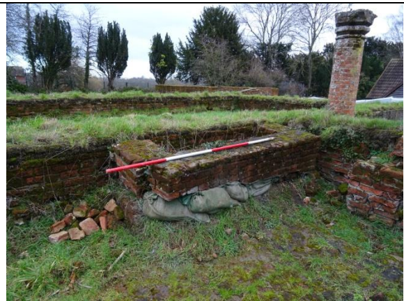
Area 1 sand bags inserted under wall
