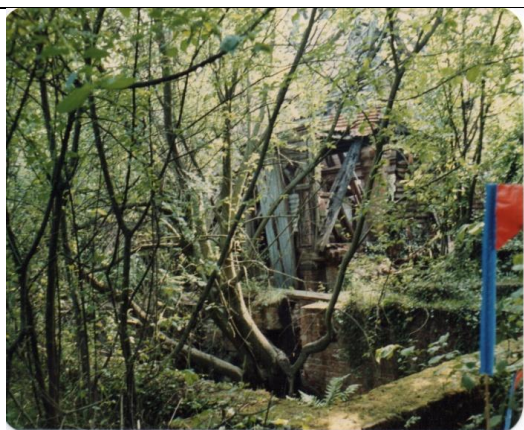
Large cellar in 1982; looking south west
