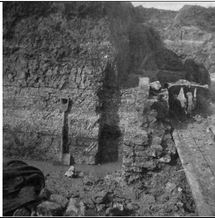
1920/30 picture of well south wall (Photograph Bromley Historic Collection)
