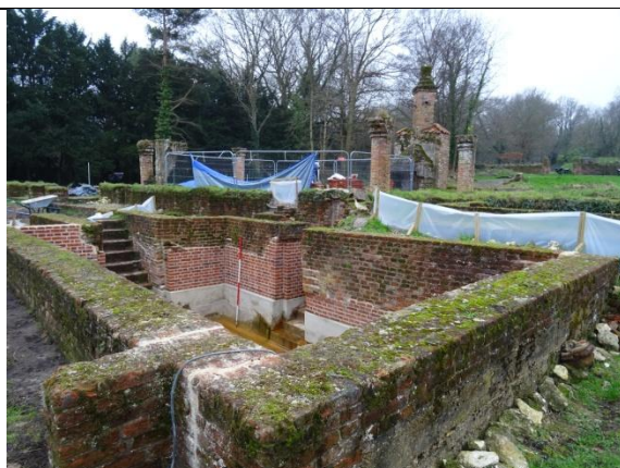
Large cellar in 2022; looking south west
