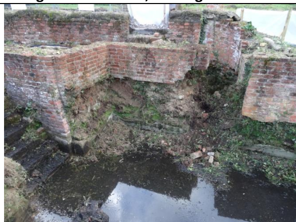
Cellar 2021 south west corner before work
