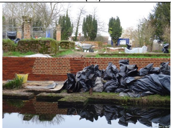
Work in progress (H-I) 2022
