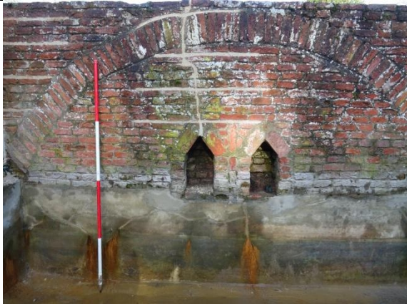
Cellar showing niches in wall
