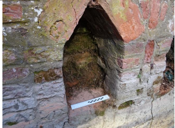
Close up of west niche
