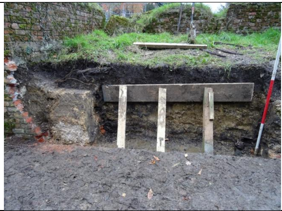
Earth bank (F-G) being supported during work
