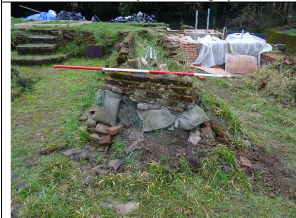
Area 1 sand bags inserted under wall
