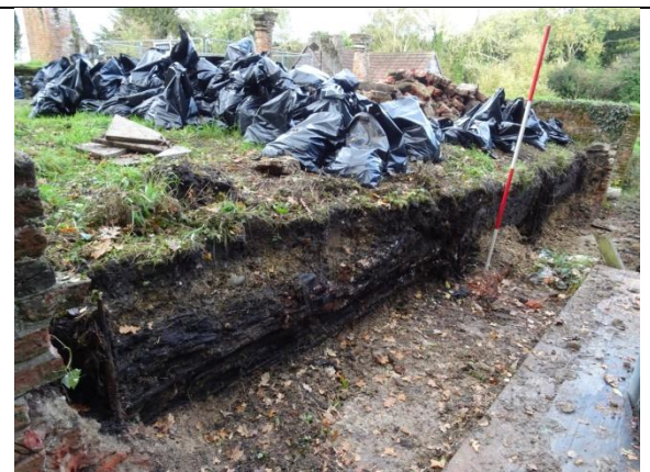
Wooden shuttering (D-E) after wall removed
