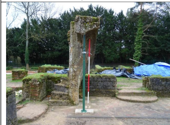
Hall; Acro Prop inserted to support stairs
