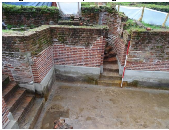
Cellar 2022; after work completed
