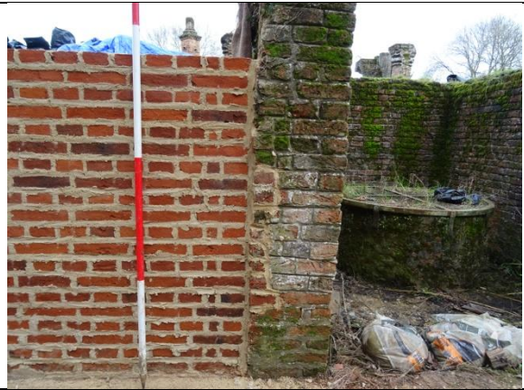
Well south wall in 2022
