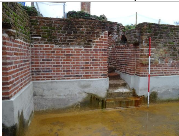
Large cellar 2022; after work completed
