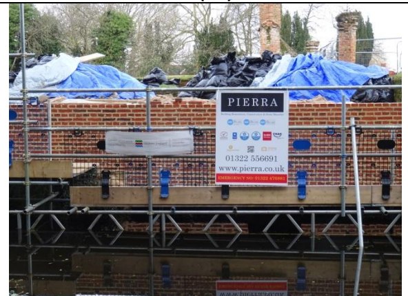
South wall (D-E) during work 2022
