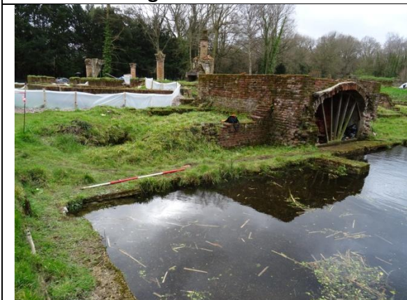
North island; sand bags inserted under wall
