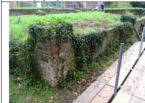
South west corner (D-E) before work 2021
