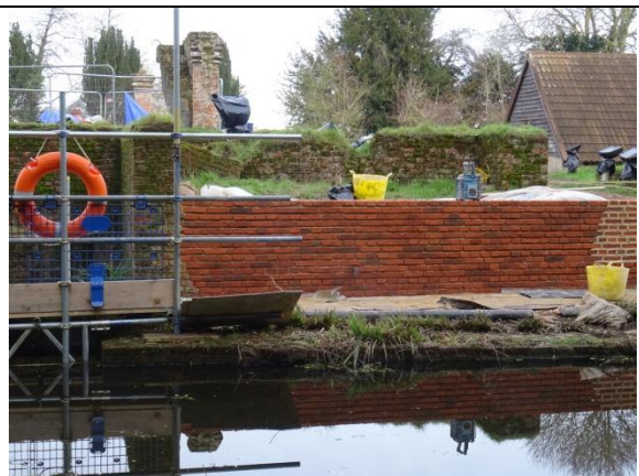
Middle of south wall (F-G) after work 2022
