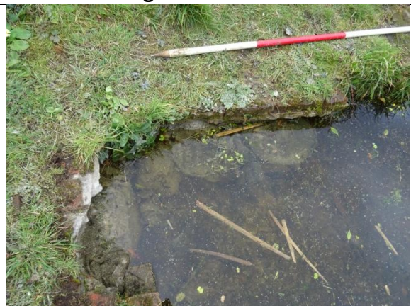
Close up sand bags inserted to support wall
