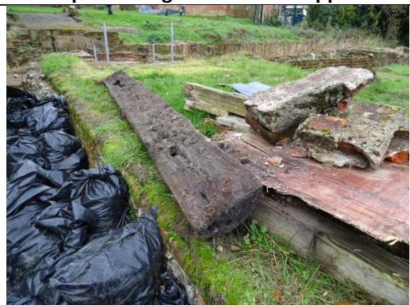
Wooden shuttering from the south wall
