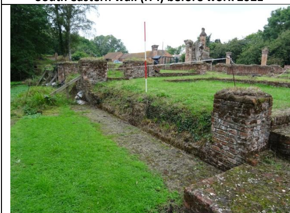
South eastern wall (H-I) before work 2021
