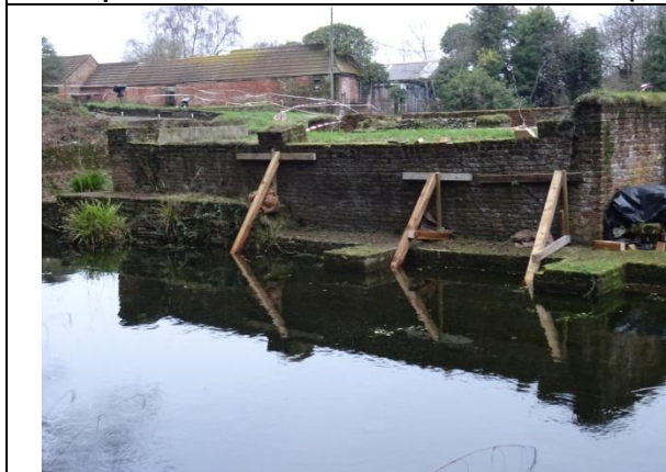
South western end of south wall (D-E) with temporary props in place before work 2021
