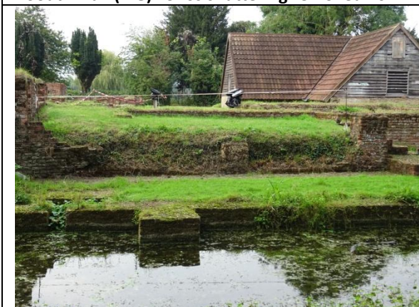
South eastern wall (H-I) before work 2021
