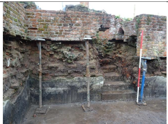
Cellar 2021 south west corner before work
