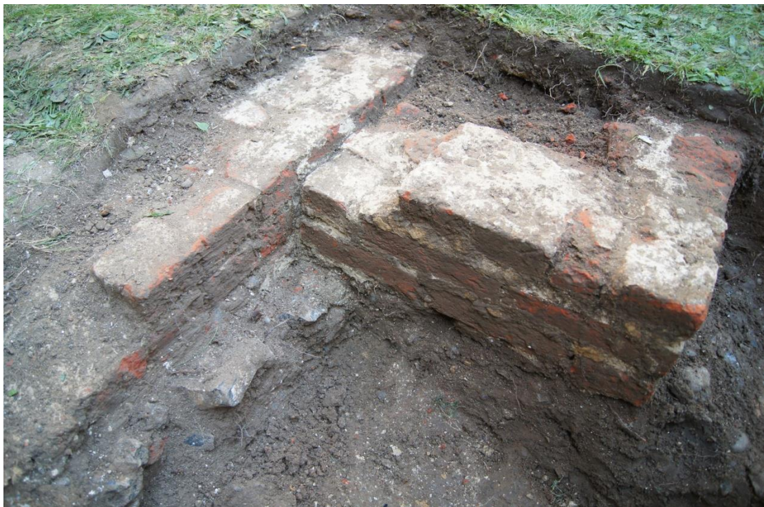
6. View of excavated foundations of presumed north wall of service pantry
